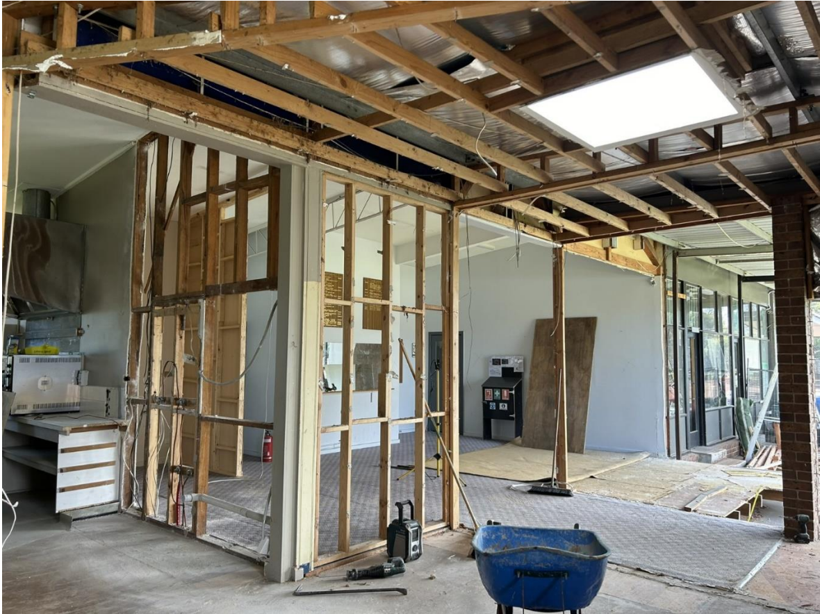
Stud walls of new RSL Remembrance Lounge July 2024
